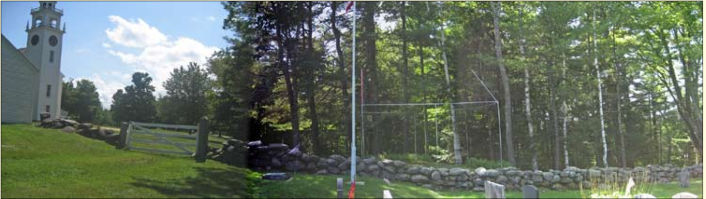
A view from the Old Burying Ground looking south with the Meetinghouse on the left and the tubular steel mock-up of the proposed Hearse House at center right. (It was moved to the west 15 feet following the Charrette on August 23rd.)
