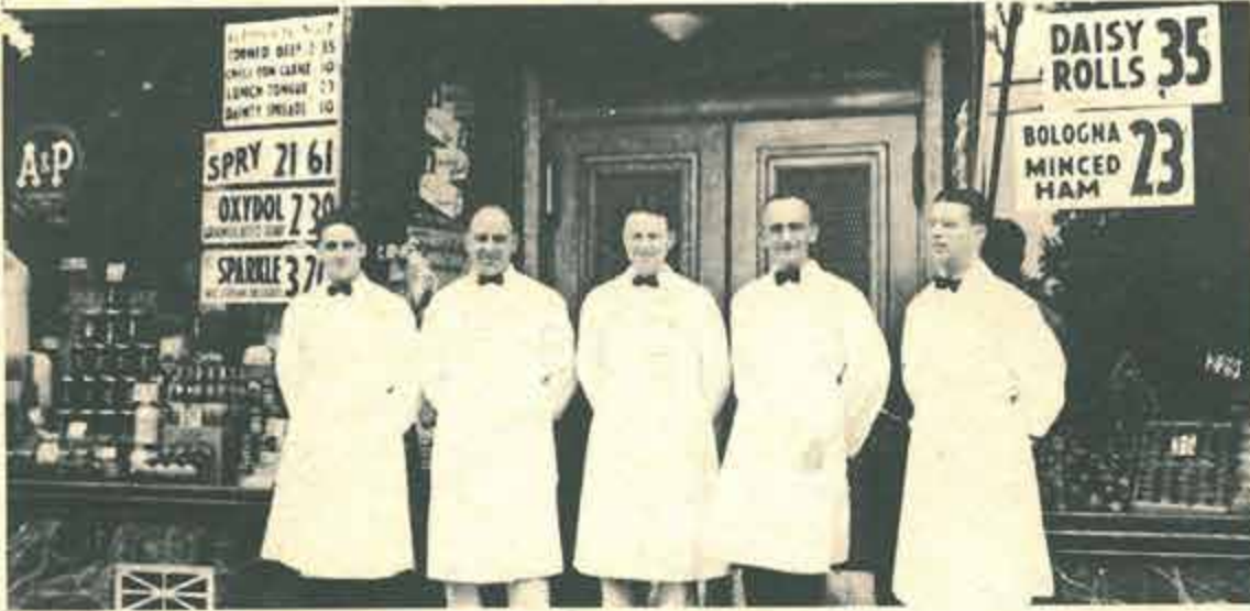
Remember the A&P on Main Street? It moved out near the end of the thirties and it is now occupied by Christie and Thomson motors. In front of the store, from left, are John Heil, Cy Young, Reglis Lessard, unidentified, and Harold Lambert.
